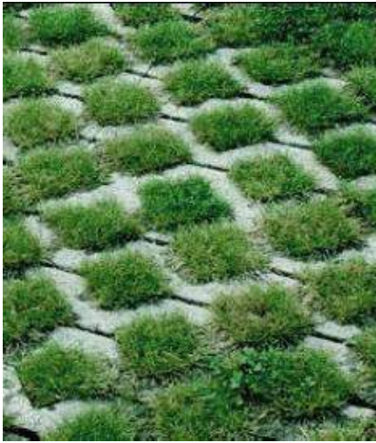
Figure 21: Passive Rainwater Harvesting Methods: Permeable paving and Rain Gardens Source: https://www.thebetterindia.com/57856/rain-harvesting-tips-india/
