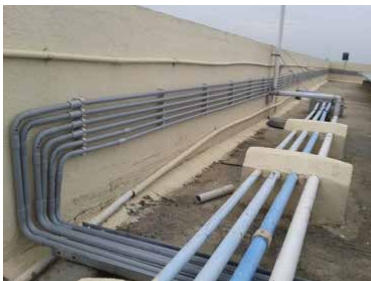
Picture 27 Proper Cable Routing in Dedicated PVC Pipes Clamped on the Wall
