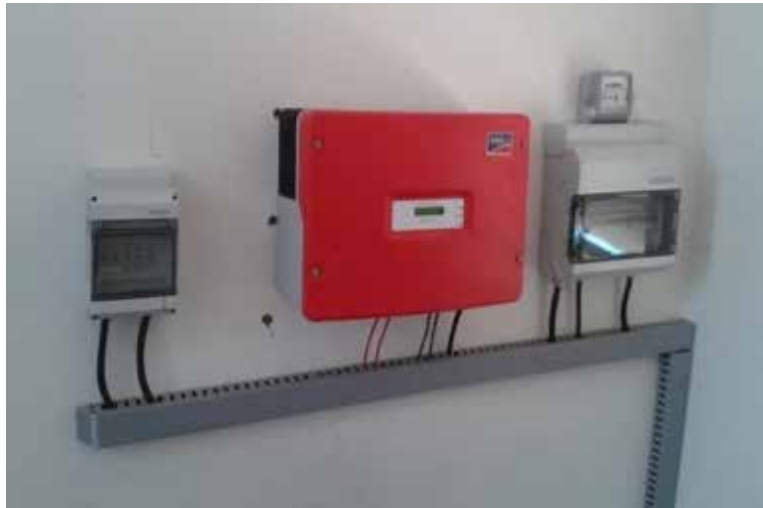
Picture 16 DC Distribution Box, solar grid inverter; AC distribution box
