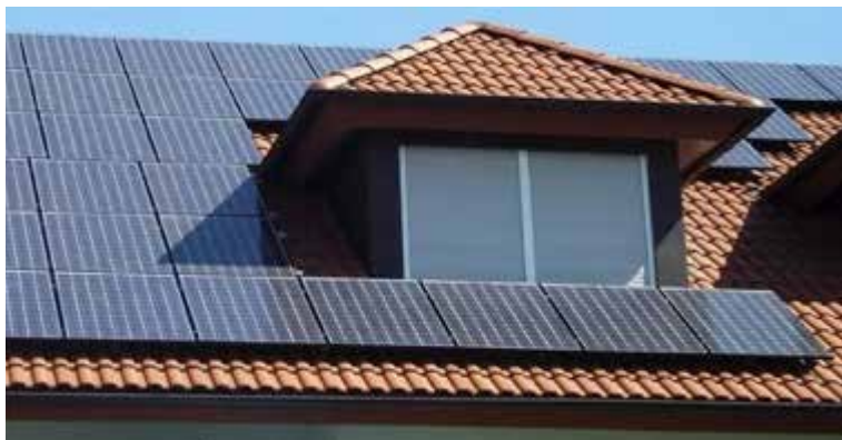
Picture 22 Design Default: Shading from the Building
