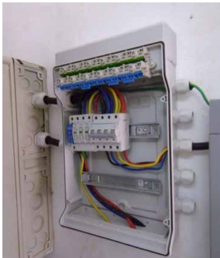
Picture 28 Proper Cabling and Connections Inside the AC Distribution Box
