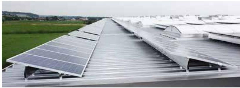
Picture 8 Professional Mounting System Attaching Directly to the Corrugated Roof Sheet
