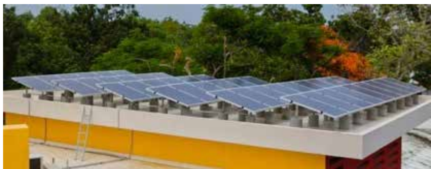
Picture 3 10 kW grid-connected Rooftop System at Auroville, Tamil Nadu
