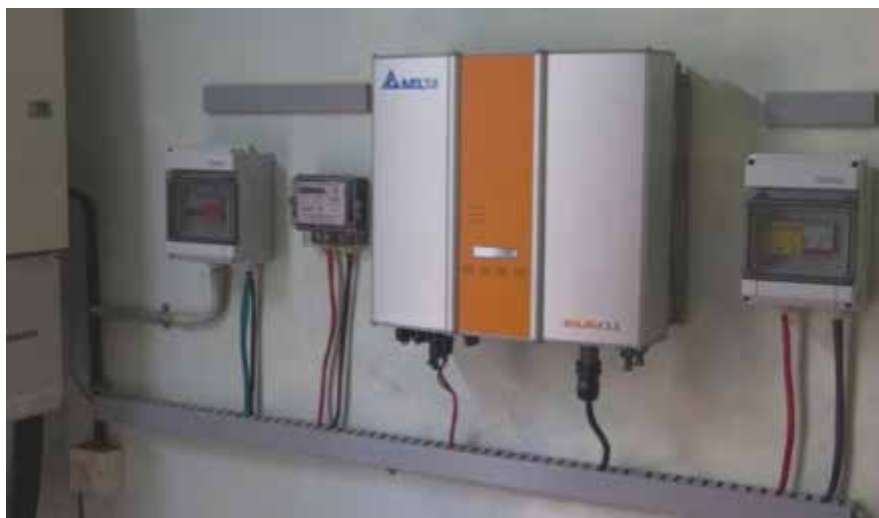
Picture 13 Solar Grid Inverter 3.3 kW Capacity
