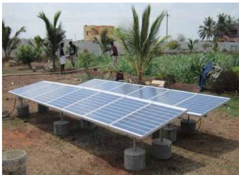
Picture 11 Ground installation with removable concrete foundation blocks
