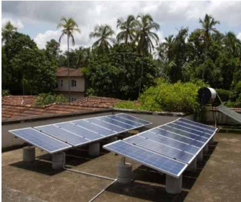
Picture 7 RCC Flat Roof Mounting with Removable Concrete Foundation Blocks
