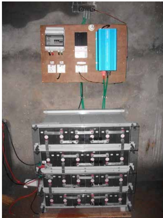
Picture 1 Stand-alone Solar system with battery pack
