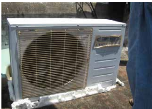
Outdoor metal cabinet of a split-system ( front view)
