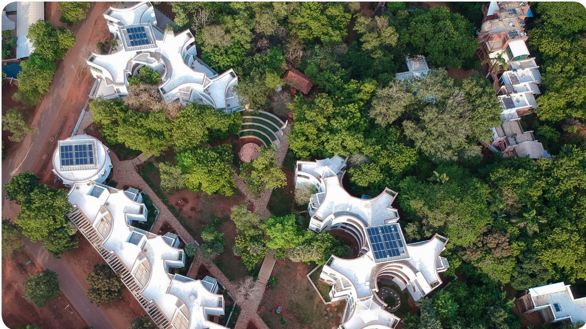
Figure 5: Rooftop Solar panels at Kalpana
